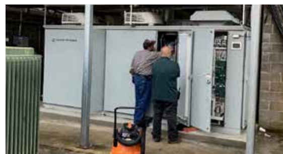
Figure 6. Old S&C static UPS with battery being replaced.
