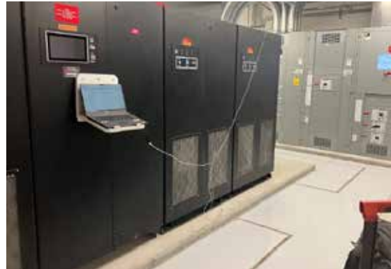
Figure 4. One of four CLEANSOURCE® XT 500Z UPS undergoing commissioning.
