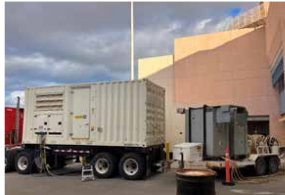
Figure 6. Wagner CAT supplied diesel generator and load bank used during commissioning.
