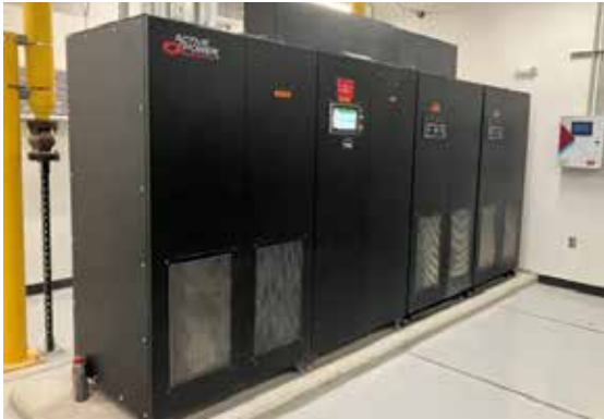
Figure 3. One of four CLEANSOURCE® XT 500Z UPS installed on a concrete pad.
