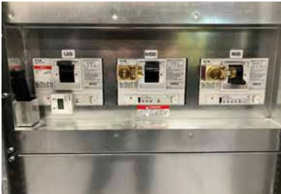
Figure 5. One of four 1000A MBP with SKRU manufactured by C&C Power supplied by Active Power.
