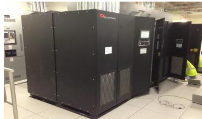
CleanSource 600 kVA UPS (N+1) being installed
